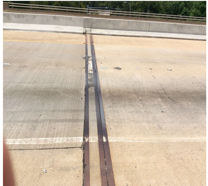
PHOTO 2 Description Bent 1. Top of backwall is breaking apart
