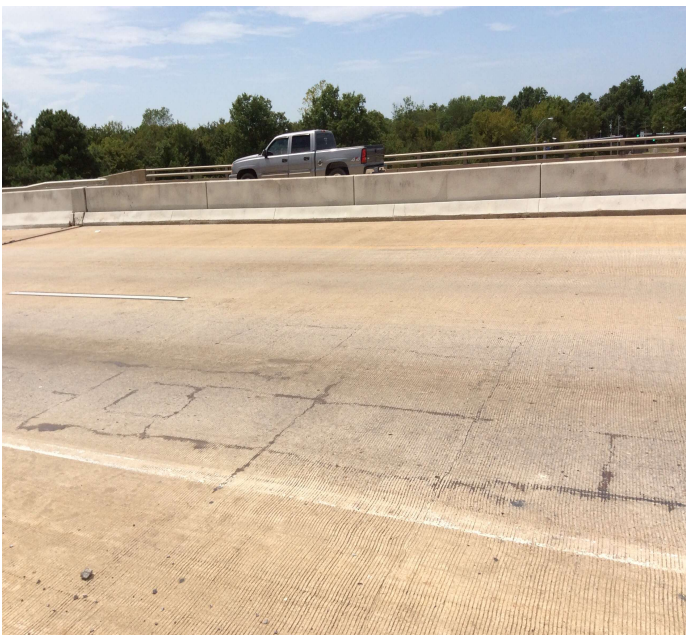
PHOTO 1 Description Unsealed cracks in the Left Lane.
