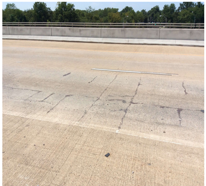
PHOTO 2 Description Right lane epoxy repairs.
